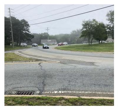
Figure 9 – Lack of pavement marking deliniating lane usage in the rotary
